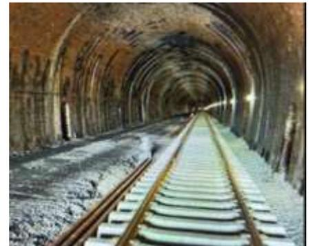
*The newly constructed test track where it passes through Dudley Tunnel*
