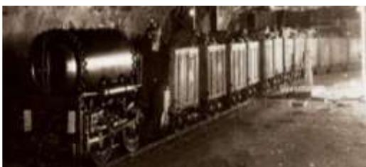
*Compressed air powered locomotive in Polish coal mine.*
