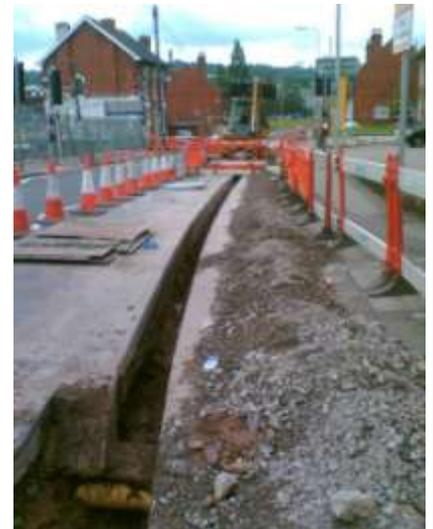
The design concept comprises a 'u' shaped sheet metal channel which houses the running rail surrounded by packing materials based on railway level crossing practice.
