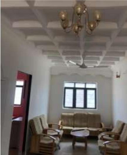
*PBP customer in Khartoum has recently sent a picture of a ceiling which is the underside of a lightweight flat roof built with the Parry 'High and Dry' waffle technology.*
