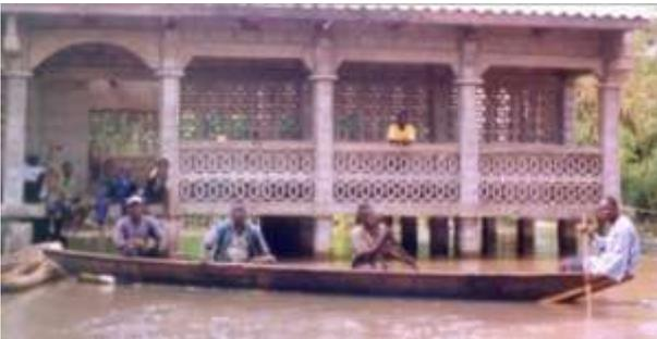
For communities prone to flooding, further development of low cost methods of building on raised columns, already tested in Benin and Mozambique
