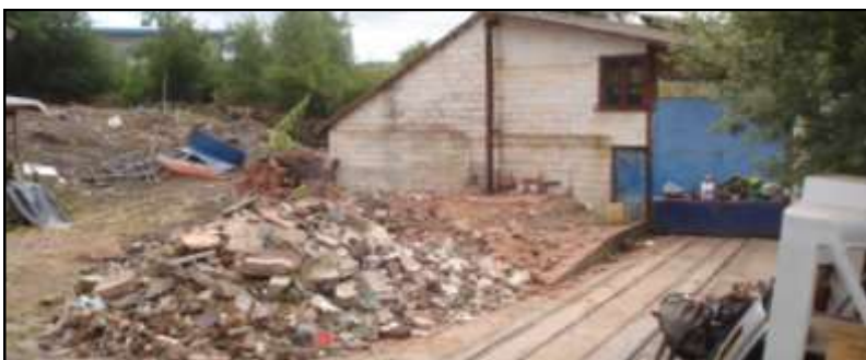
An important example of Intermediate Technology innovation reduced to rubble while also rendering inoperable the narrow gauge railway.
