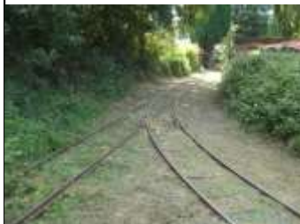
600mm gauge line with 70v charging points for flywheel - powered rail vehicles blocked
