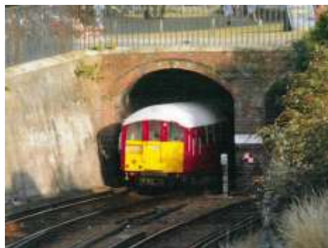
Headroom to spare, Island Line train (ex LUL stock) emerges from tunnel.
