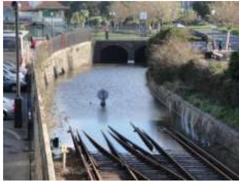
The approach to Ryde Tunnel entrance temporarily inundated. Services suspended electrical equipment damaged
