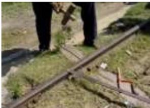
The railway's own permanent way gang were perfectly able to put the track right using simple equipment. With track workers earning only £2 a day, a couple of gangs providing continuous attention to keeping the track straight will barely affect the railway's operating costs while greatly improving safety and efficiency.
