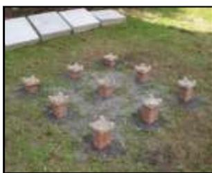
**Simple stilts, using pairs of bricks embedded in ground**
