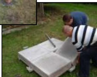
Experiments are in progress producing precast units, light in weight so as to be convenient to manhandle which assemble into a complete floor.
