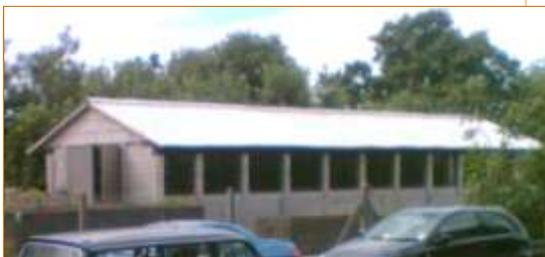
***Railcar depot design suitable also for use for warehouses for agricultural produce such as coffee beans, tea, rice or sorghum. The Stourbridge building provides a covered area of 160m<sup>2</sup>. In a developing country it could be built for less than \$20,000.***
