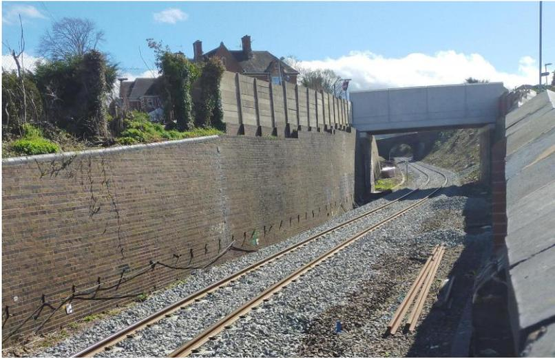
Many of the smaller and most remote lines of the UK rail network have for years only received 'patch-and-mend' maintenance and still comprise of extremely old materials dating back decades. As a result of historic wear and tear, these lines have rails that have become distorted. Where the ends meet, there is often a 'drop' or 'step' causing impact damage and noise as the train wheels pass over the uneven joints.
